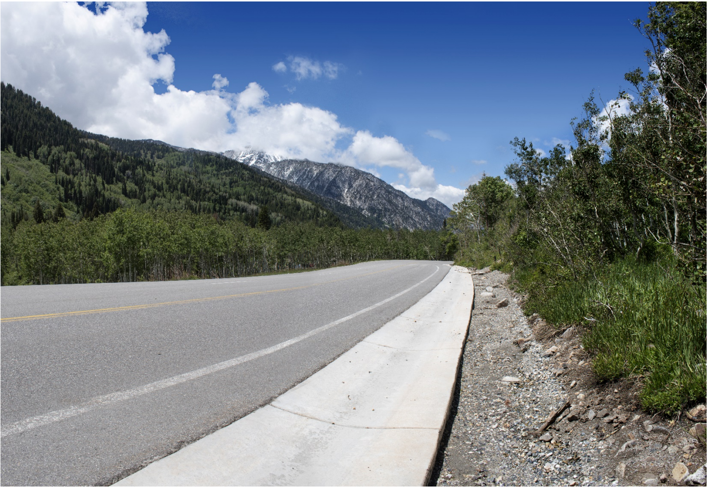
KOP 16 – Existing Condition – White Pine Trailhead
