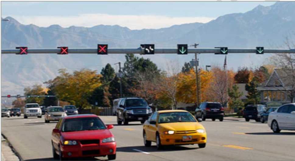
Figure 2-7. Changeable Lane-control Signals
